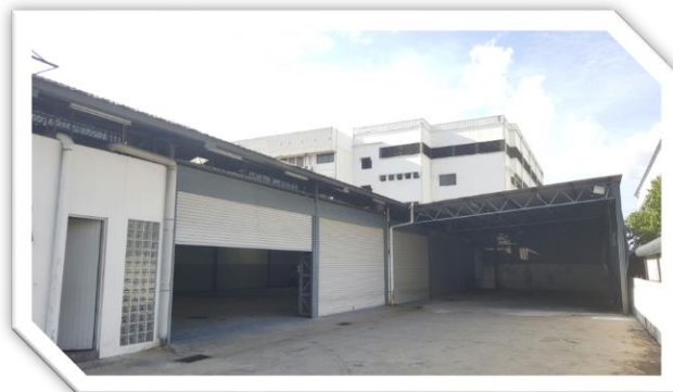
Warehouse and Production Facility in Petaling Jaya, Malaysia
